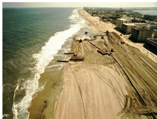
Figure 4: Soft Coastal Defense Structure (Nourishment)
