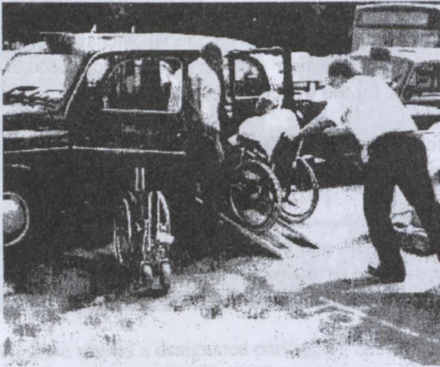
Figure 9 shows a London Taxi cab with makeshift ramps. This design does not allow for independent entry. 3
