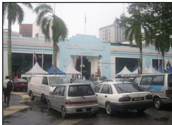
Fig. 1.0: Case Study 1-Central Market Building
