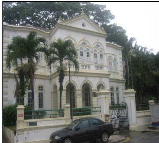
Fig. 2.0: Case Study 2- PAM Centre Building
