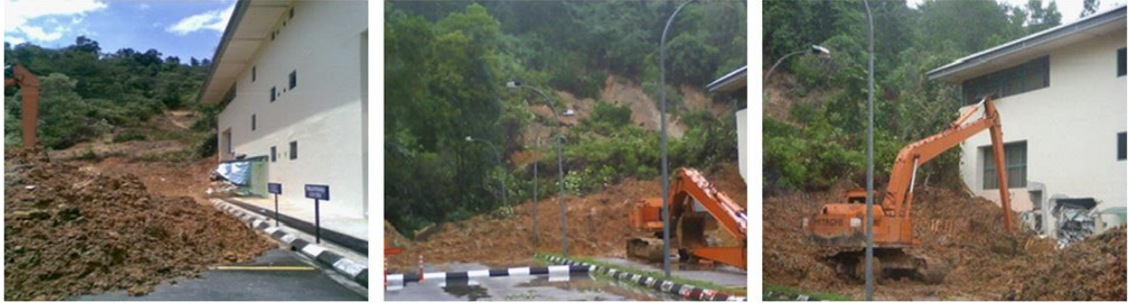
Fig. 1. Landslide area and clearing works in progress.
