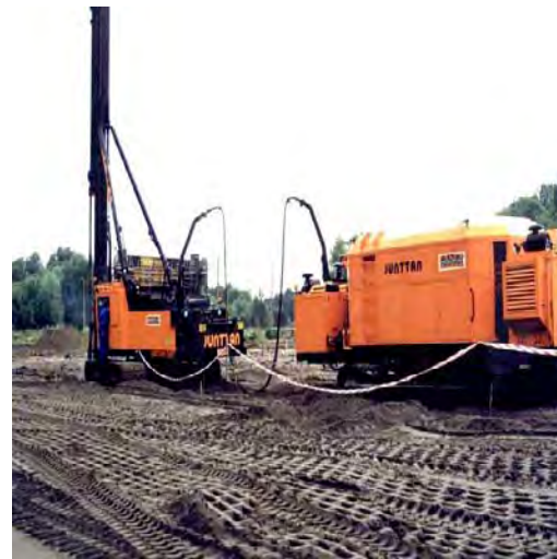
Figure 2: (a) Deep wet mixing plant with (b) separate mixing and holding tanks and pumps.
