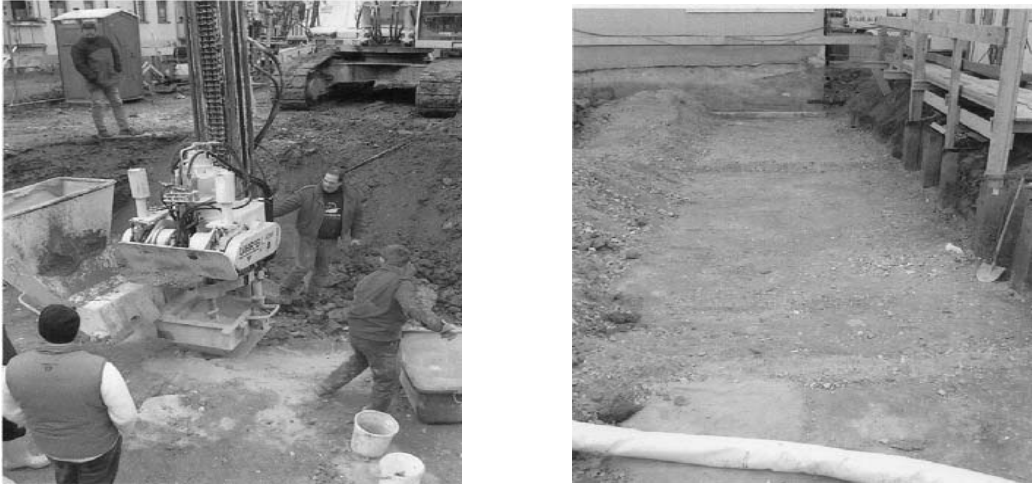
Figure 6: (a) Installation of the CSV-columns, (b) Work plane after CSV installation
