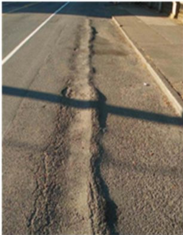
Figure 5. Permanent deformation in asphalt pavement.
