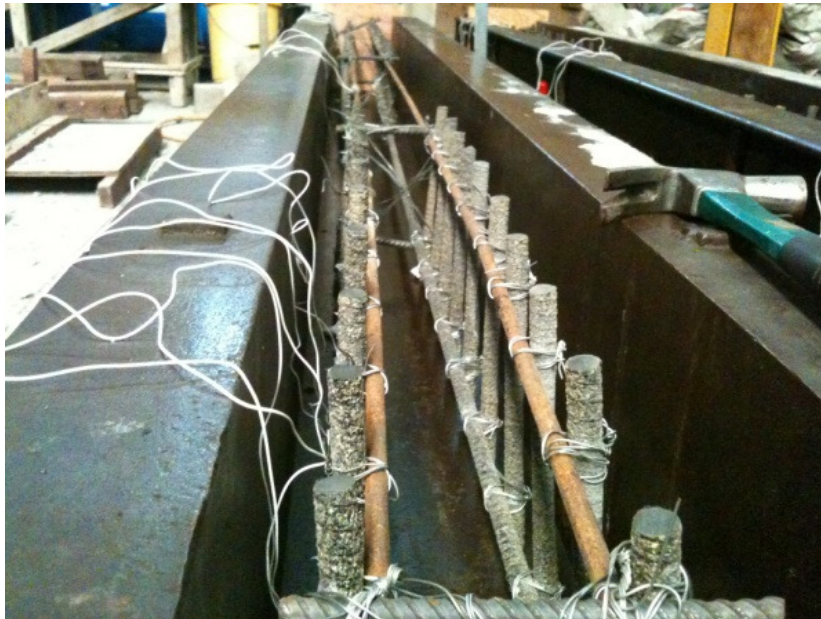
Figure 5. Beams in moulds to cast.
