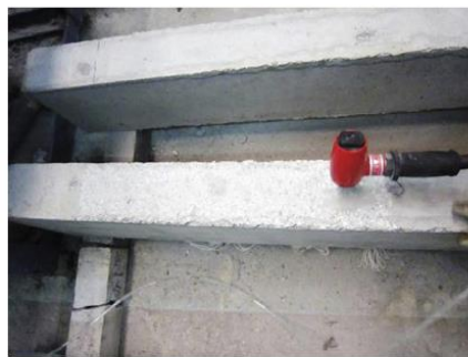
Fig. 4. Surface preparation of the concrete beam.
