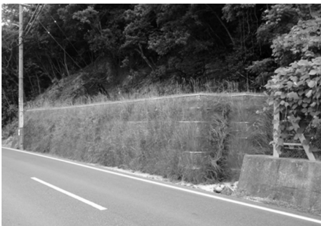
Fig. 1. Application to a rockfall protection wall.
