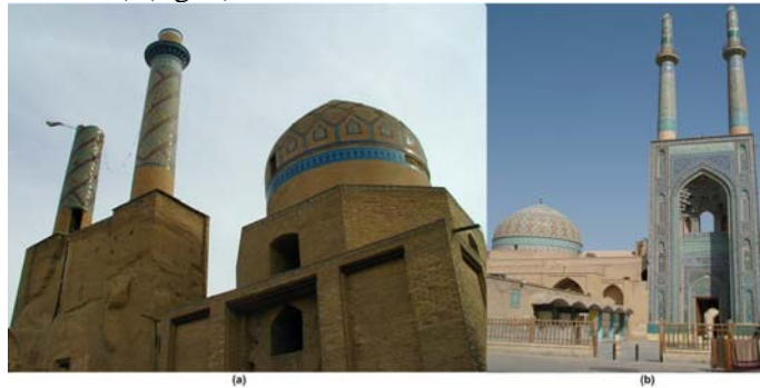
Figure 5. a) The discontinuous double-shell dome topped the Sultan Bakht Aqa mausoleum in Esfahan; b) The continuous double-shell dome of the Friday mosque in Yazd. (Source: Authors)
